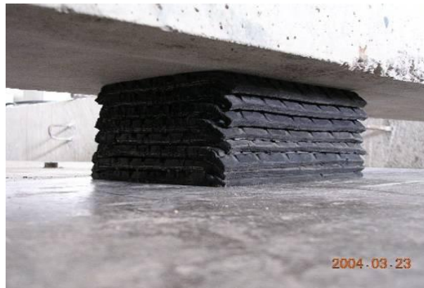
Fig.16 Scrap tyre pad as low cost isolator device.
