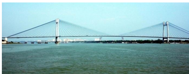
Fig 4: Vidya sagar setu at kolkatta used tmt bars for construction
