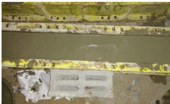
Fig 3.2 Casting of beam
