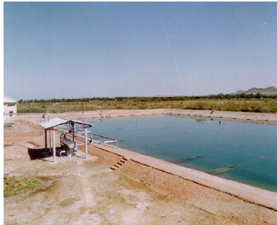
Fig.2 Solar pond at Bhuj
