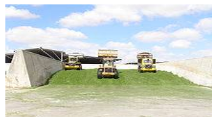
Figure-2: bunker image
