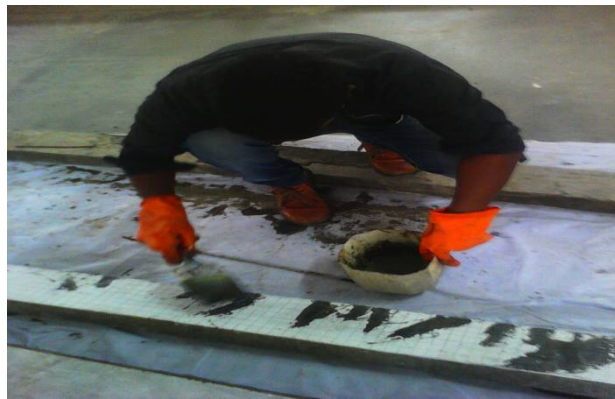
Fig. 2 During Repairing Of Beams By Using Epoxy Bonding Agent
