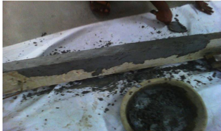
Fig. 3 after applying of super latex with beams
