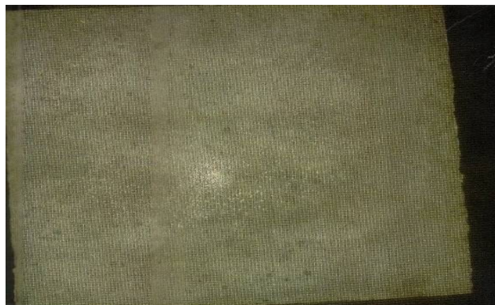
Fig no. 5 Precipitation on Surface of Concrete Cube.
