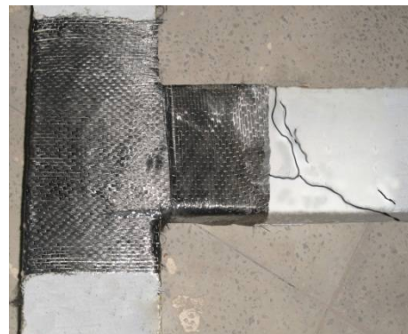
Fig. 9. Crack Pattern of BCJ CF-02
