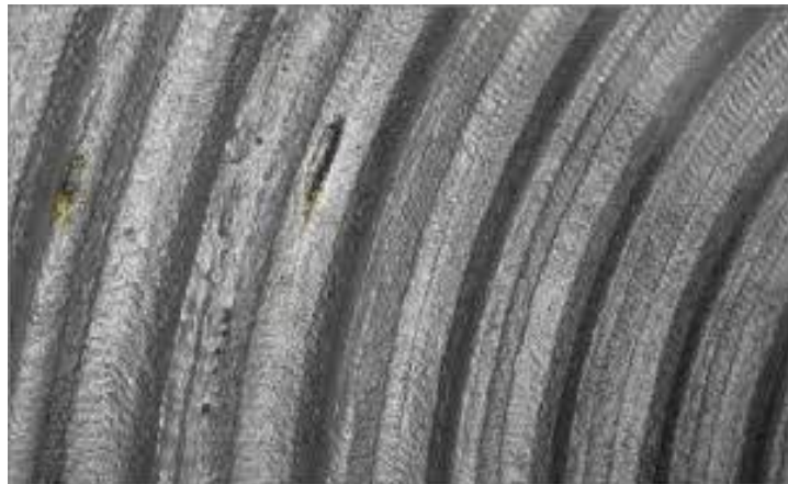
Fig. 3.5 weld overlay coating
