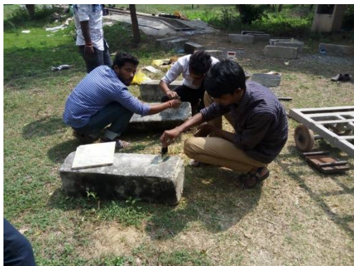
FIG1.2.EPOXY INJECTING ON CRACK
