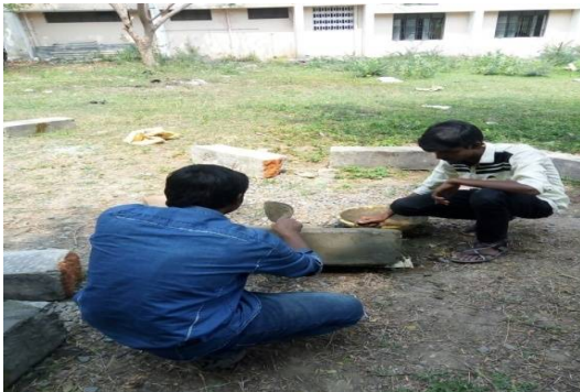
FIG.1.4 MORTAR APPLIED ON THE BEAM
