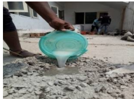
Figure 4.3 Adding solutions to the binder and aggregate mixture
