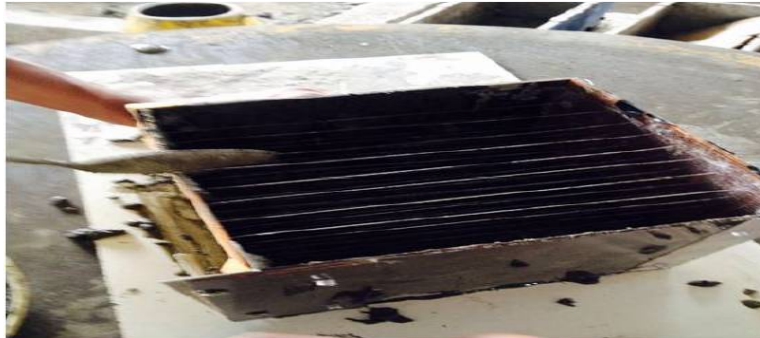
Fig 3 Pouring of cement concrete
