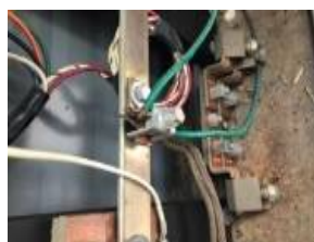
Improper grounding
