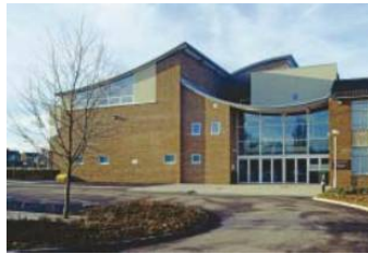
Fig. 1. sample attached for evaluation (a) The new entrance (b) Master plan (c) section
