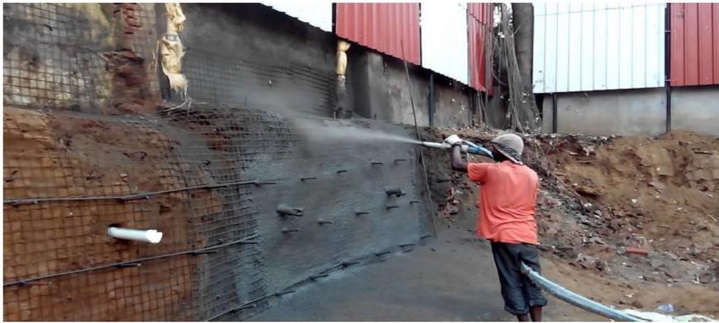
Figure 1.3 shows the pneumatically applying concrete on repair surface
