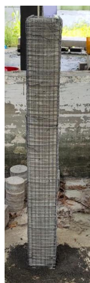
Fig-2 Column with double layer of weld mesh
