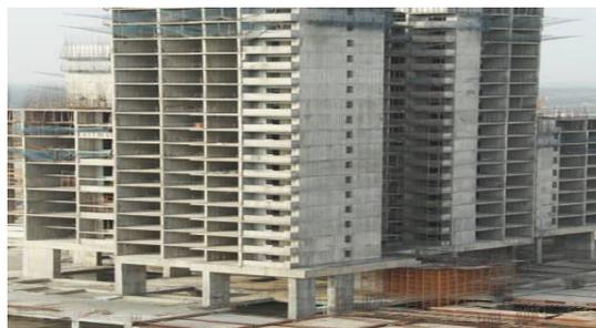
Figure 1:- Transfer slab With Shear wall
