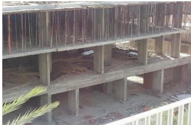
Figure 2:- Transfer slab With Column
