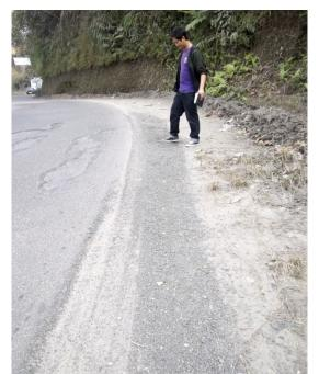
Figure 6. Total edge raveling failure- can cause accidents in case a vehicle take over from extreme corner as it's located on S-curve.
