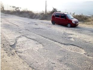
Figure 1. Pot holes and longitudinal cracks
