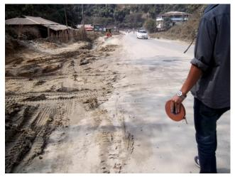
Figure 8. Mud on road side-Yupia. Not recommended as it reduces skid resistance of vehicles causing slipping
