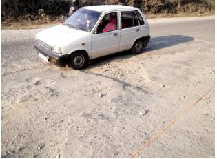
Figure 2. Deep pot hole consuming almost half of wheel radius (175mm deep)
