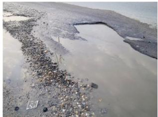
Figure 5. Big pot hole filled with drainage water and raveled aggregates (Naharlagun)
