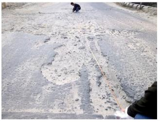
Figure 7. Total failure of pavement in Nirjuli
