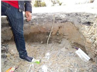
Figure 9. Failure on road side caused by subgrade failure
