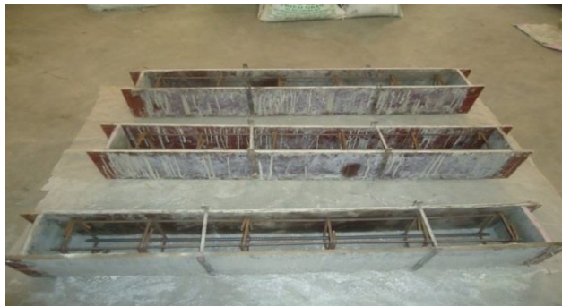
Figure 5: Formwork
