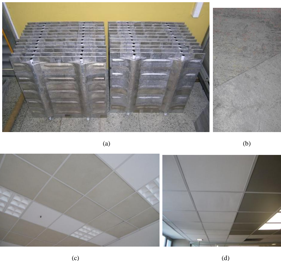
Fig. 1. Ceiling heating/cooling panels made of aluminium foam developed by IMSAS (a), example of their surface design using thin-walled composite surface foil with trade mark MWM Design – Clasic Stone produced by German company MWM GmbH & Co KG, Arnsberg (b) [2, 3], installation of aluminium foam panels in SmartGrid laboratory of IMSAS in Bratislava (c) and in the open office space area 260 m 2 of company Sapa Profily a.s. in Ziar nad Hronom, Slovakia (d).
