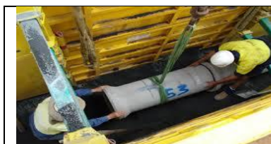
Fig 1.1 Geopolymer concrete sewer pipes being installed in Toowoomba, Queensland, Australia.(2005)
