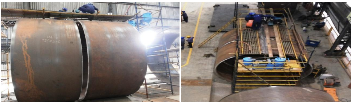
Fig-1 Existing platform for SAW welding
