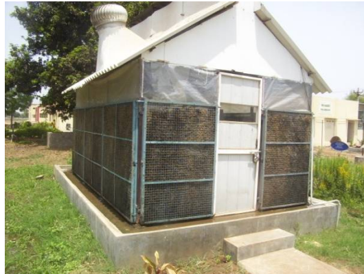
Figure 1: On-farm evaporatively cooled storage structure
