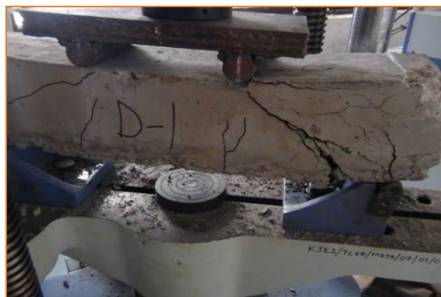
Fig. 7 Shear cracks for C beam
