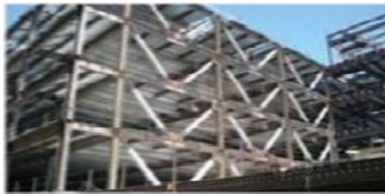
Fig2: Braced tube structure
