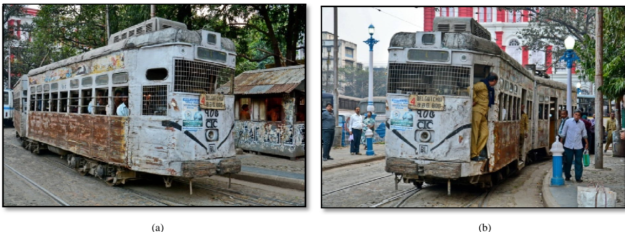
Fig. 2. (a) Old modelled tram bus and undulated pavement (b) Improper stoppage to ride the tram. (Source: www.flickr.com/photos/asienman )
