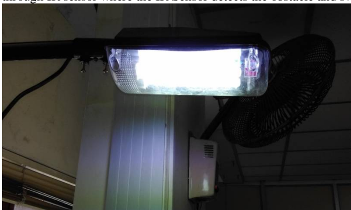
Fig 7.5: Status of the Light is ON after obstacle detection
