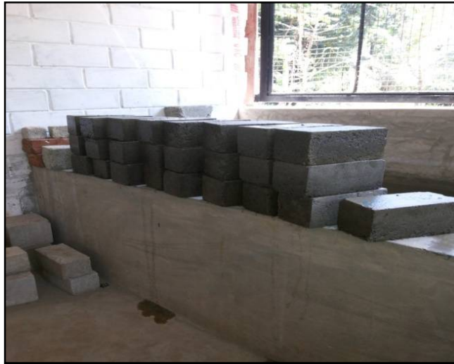
Figure 3. Prepared solid concrete blocks after curing
