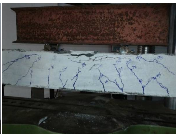
Figure 3: Crack Distribution At Failure Load.
