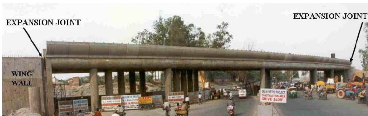
Fig.5:-Flyover using integral bridge concept for Delhi Metro (the curved flyover has no bearing or expansion joints on piers/abutments; length: 115 m)
