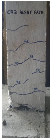
Fig. 7(c). Flexural cracks in CB2
