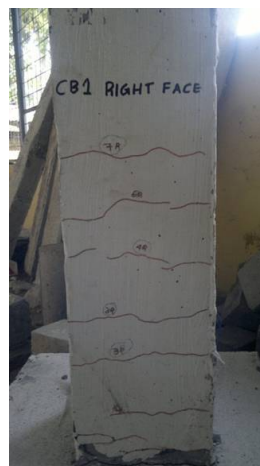
Fig. 7(b). Shear cracks in CB1
