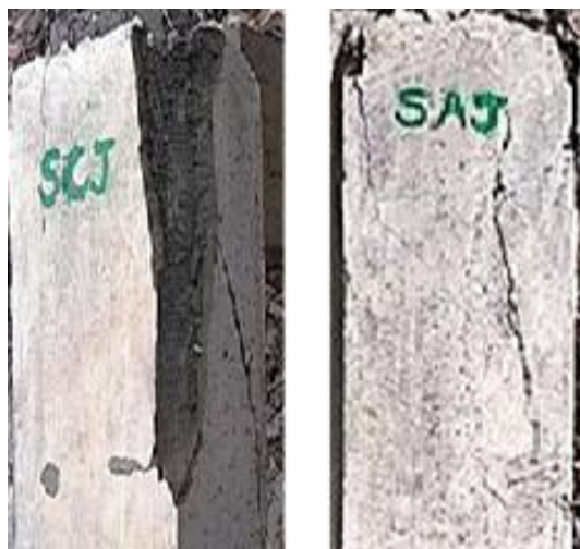
Fig. 5. Failure patterns of fully jacketed specimens
