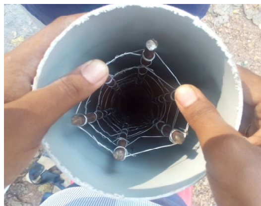
Figure 1. Reinforcement arranged inside PVC pipe
