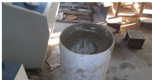
Figure 2. Column concreting using Hollow GI pipe
