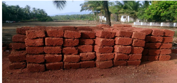
Fig. 1. Laterite blocks.
