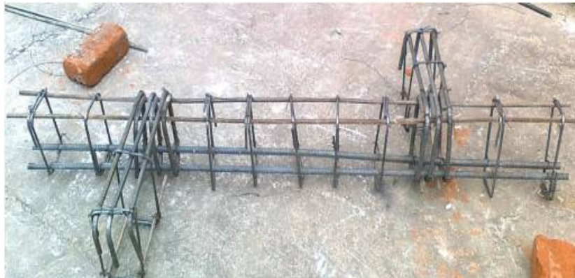
Fig.5 Reinforcement Cage
