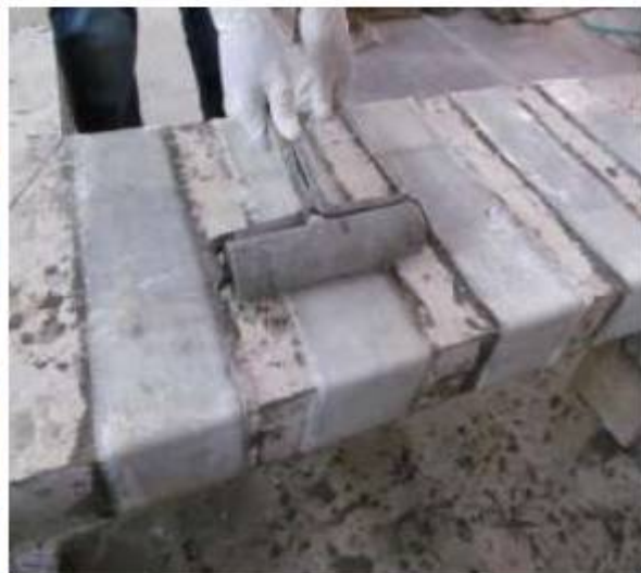
Fig. 2 Roller used for the removal of air bubble
