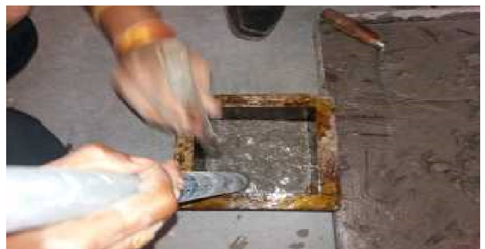
Fig. 1.4 Pouring and tempering of concrete.
