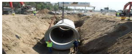
Figure 1.1 Underground Sewerage System –Laying pipes
