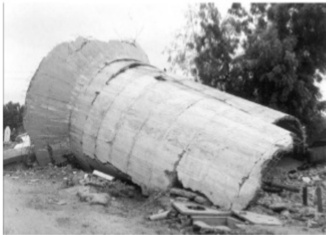
Fig. 1 Collapse of water tank in Bhuj
