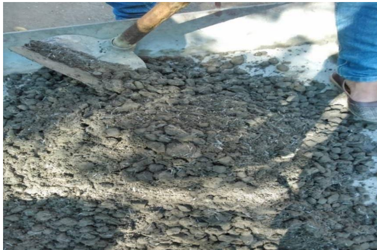
Figure 2. Dry mixing of all material
