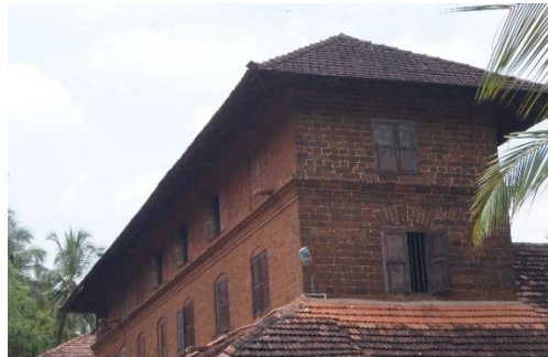
Fig 9. Exposed Laterite stone masonry
