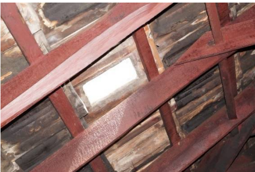
Fig 13. Top lighting using glass roof tiles
