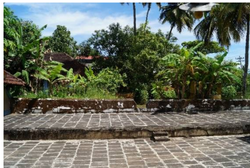
Fig 10. Unfinished granite stone flooring
