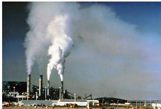
Figure 1: Industrial air pollution
