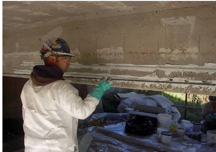
Fig. 1 Flexural Strengthening of RC Girder Source:www.aslanfrp.com
