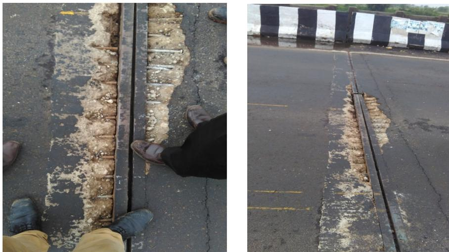
**Fig. 2: Condition of Expansion Joints showing lack of supervision during Installation**
