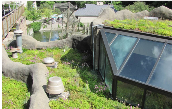
A green roof over an exhibit at the John Ball Zoo in Grand Rapids
