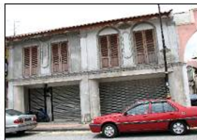
Old Shophouses building
