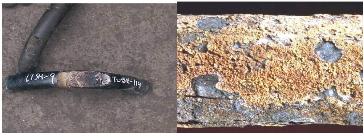
Fig 1.1 Erosion on Metal Surface
