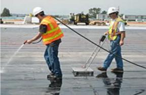
Figure 4. Low voltage platform in action
