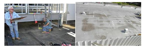
Figure 11. Nuclear meter (yellow) and grid pattern on roof
