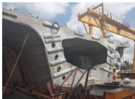
Fig 1: Casting of box girder
