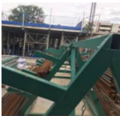
Fig 6: Cut and bent rebar storage rack.
