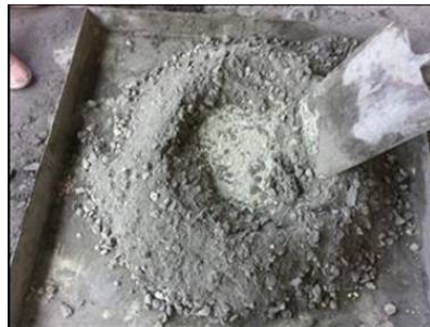
Fig 6 Concrete mixing
