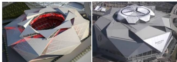
Fig. 14 Mercedes-Benz' stadium in Atlanta as an example for transformable building Source: https://www.inhabitat.com/atlanta-falcons-new-stadium-uses-kinetic-architecture-to-retract-rose-petal-roof.
